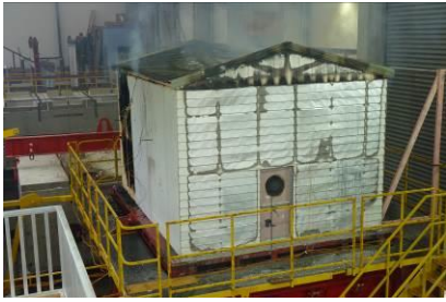
Experiment on the post-fire stability of external walls
